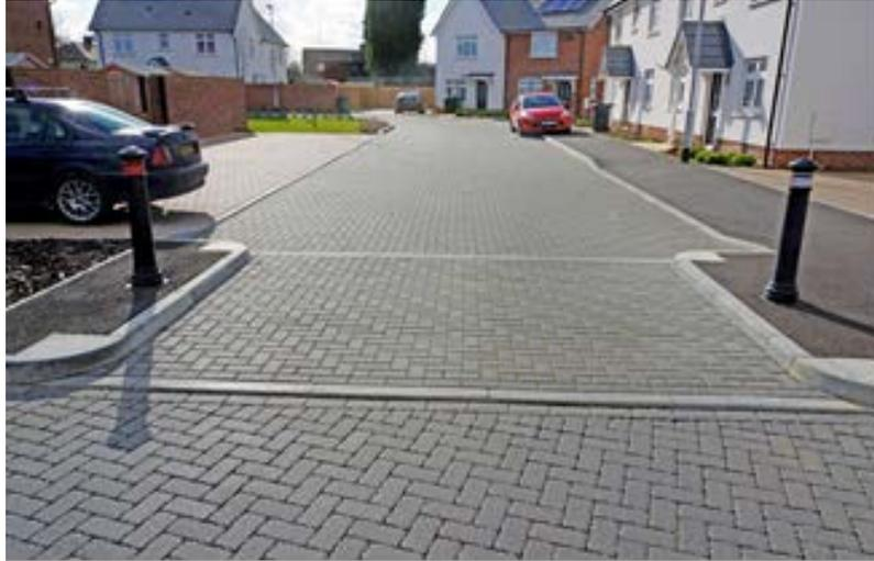
The design of permeable paving can vary significantly depending on the proposed use of the surface. Guidance should be sought from the manufacturer of the chosen permeable paving.
