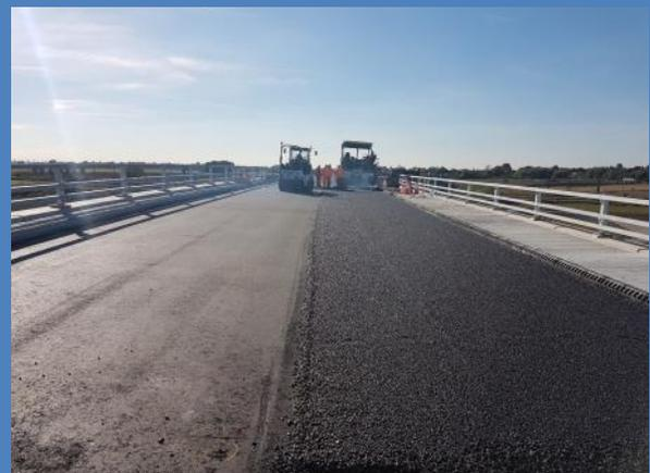
Picture right: surfacing work on the viaduct
