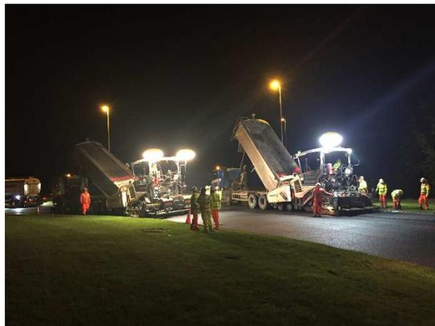
Where applicable in the package we will be using two pavers at once, instead of the conventional one machine approach. This allows us to eliminate the centre joint on the road. As joints are one of the main points of failure on carriageways if they fail or open up over time, by eliminating the central one our roads should last longer.
