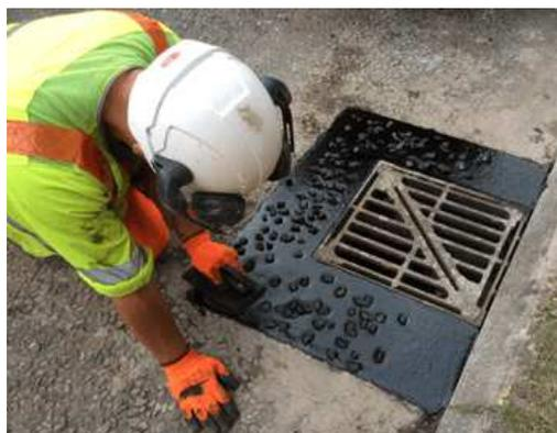
When repairing any ironwork which is likely to be overrun by vehicles, instead of following a traditional approach, we will instead be using a product called Pacopatch. The process involves patching around the ironwork in question with a polymer modified material, and resetting the gully or chamber on a more flexible bed. This allows it to resist wear and tear from continuous vehicle overrun. This is an approved system which comes with a 5yr warranty from the contractor.
