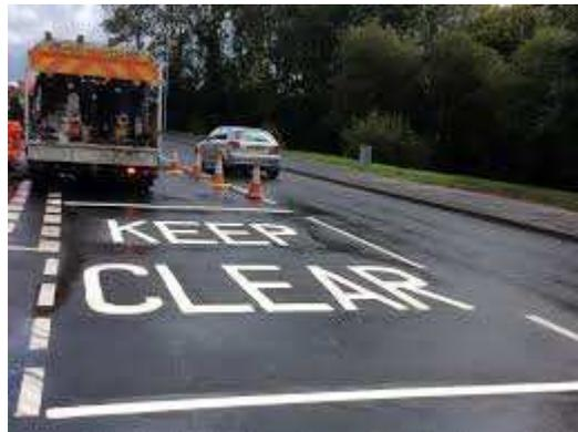
Instead of traditional road marking materials we will be using a different product called MMA. This lining material is more durable and longer lasting than normal thermoplastic, and will ensure we have to revisit site less often to refresh and renew road markings. It has a higher initial cost, however this is largely offset due to the quantity of lining required over this package, with any other differences negated by reduced future visits to redo the markings.
